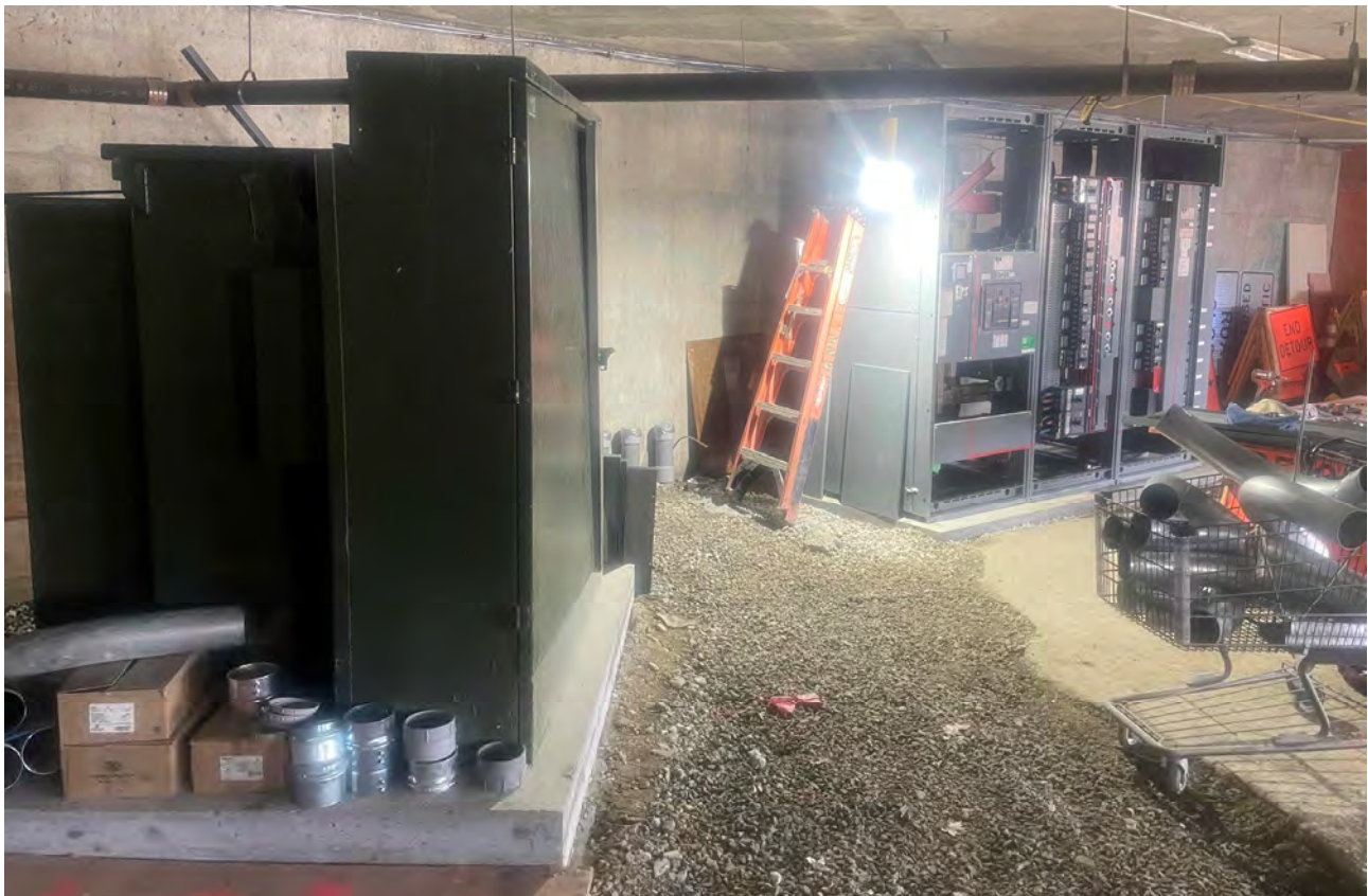
Temporary electrical service installation, in garage.
