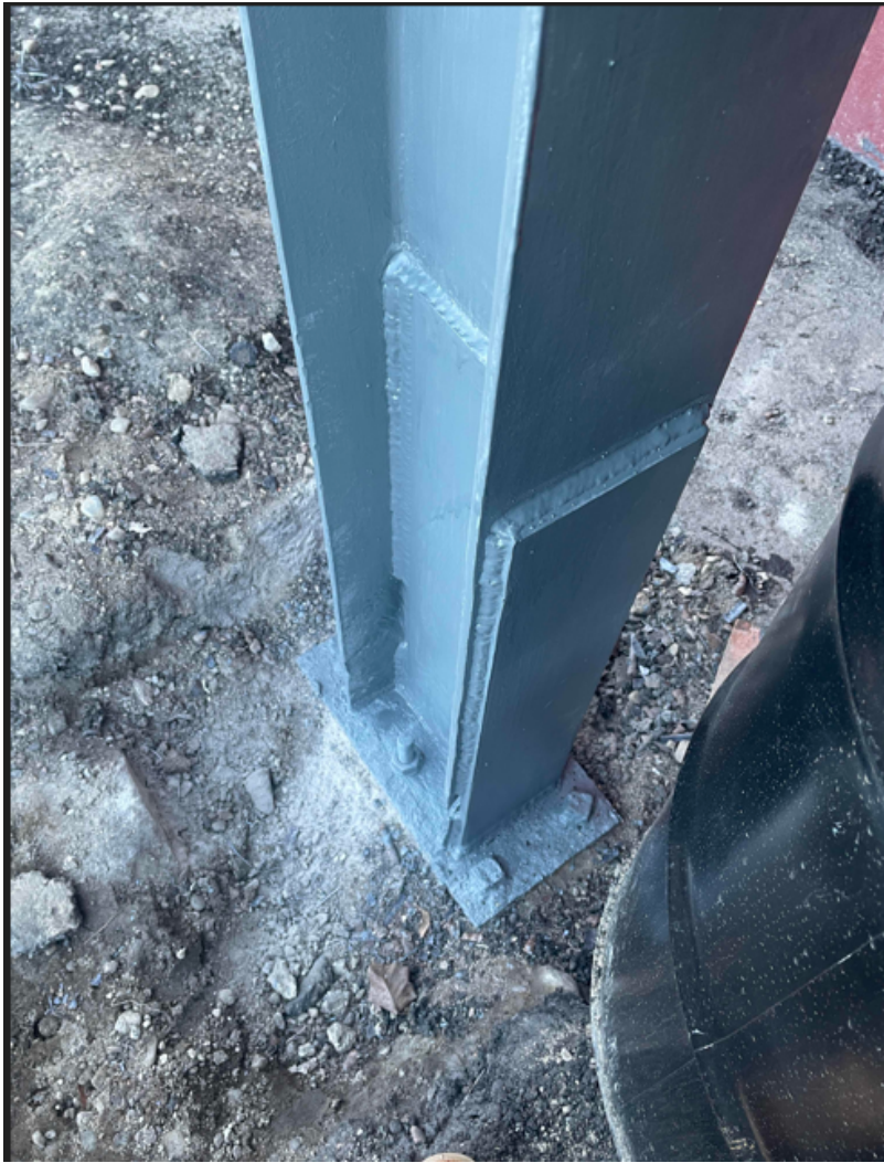
REPAIRED COLUMN 1 (2nd column from Harvard St.)
