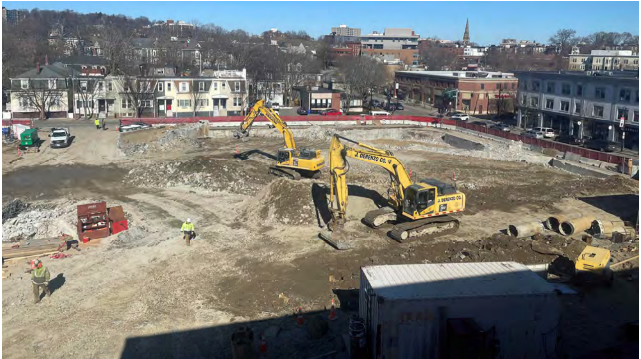
View of site, Area A, beginning of March. Foundations still in place, drilling piles.
