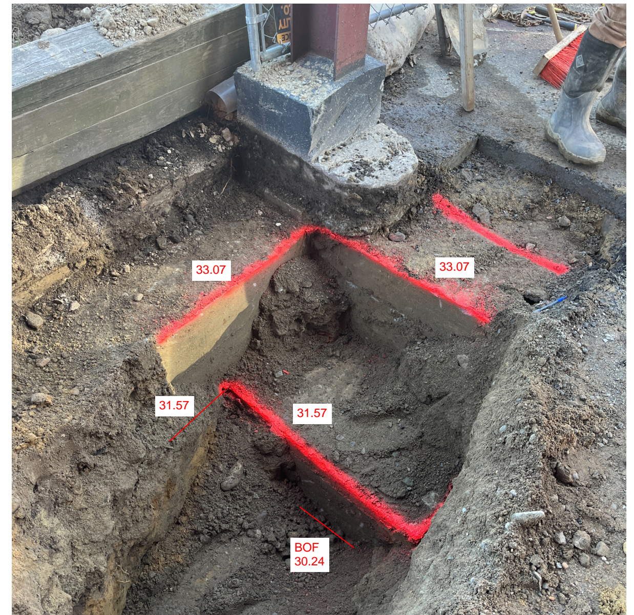
EXISTING COLUMN 2 TEST PIT (closest to Harvard St.)
