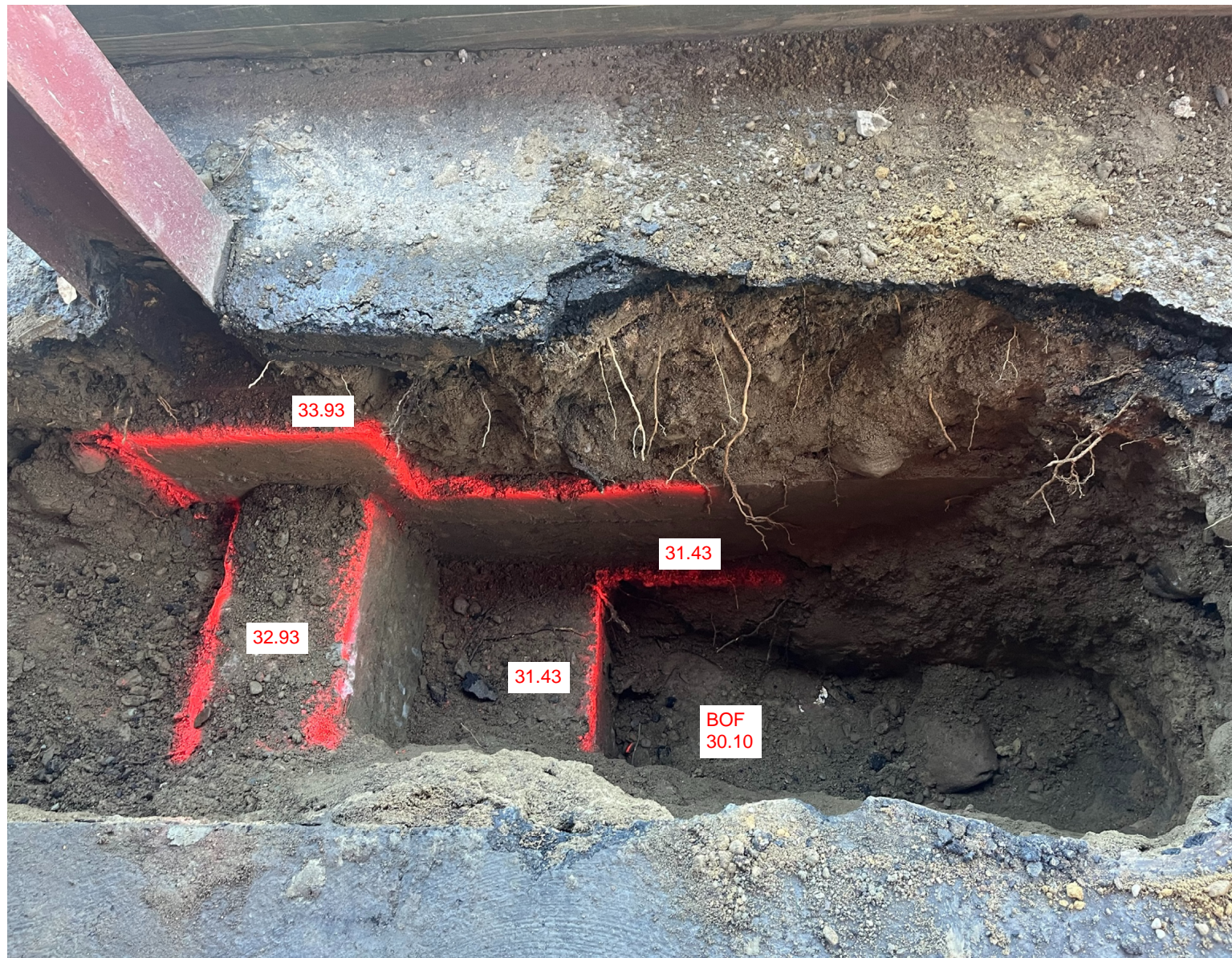
EXISTING COLUMN 1 TEST PIT (2nd column from Harvard St.)
