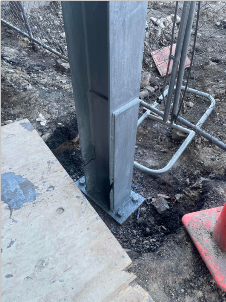
REPAIRED COLUMN 3 (3rd column from Harvard St.)
