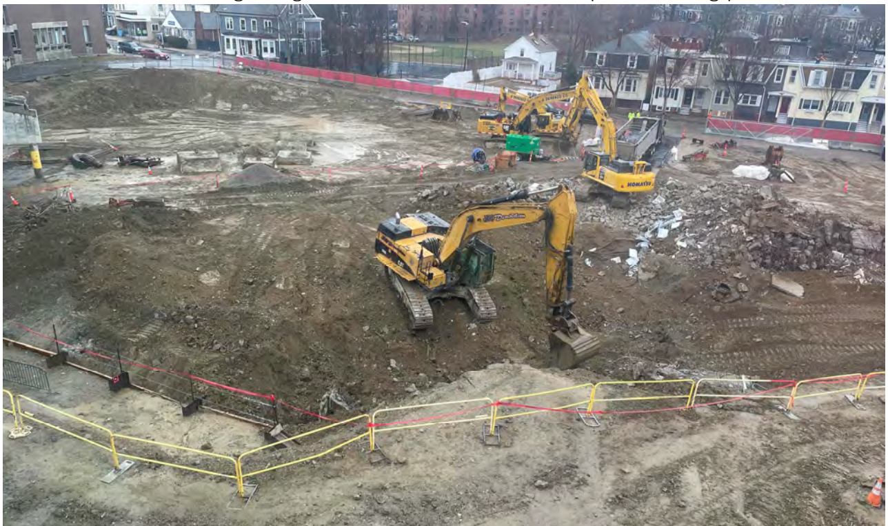
View of site, Area C, end of March. Foundations removed, lagging in place.
